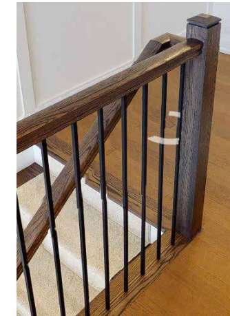
Railing Railing Package #3
